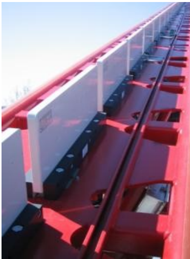
Picture 4: stators mounted on a track structure
